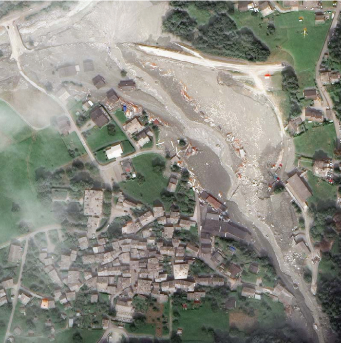
27 August 2017. Bondo after two landslides. WorldView-3. EUSI
