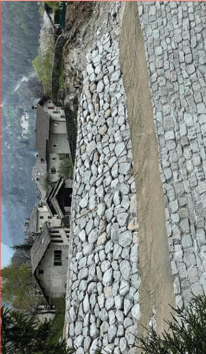
The stones of the Piz Cengalo are crushed at the nearby landfill and then installed. (Photo: Hanspeter Schless)
