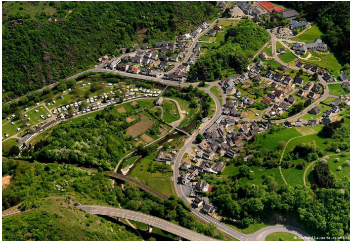
Condition before the flood disaster.
