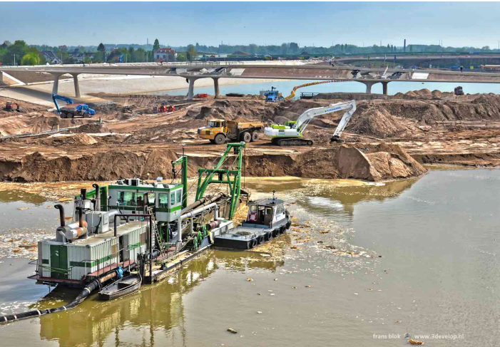
Construction of a new channel.
