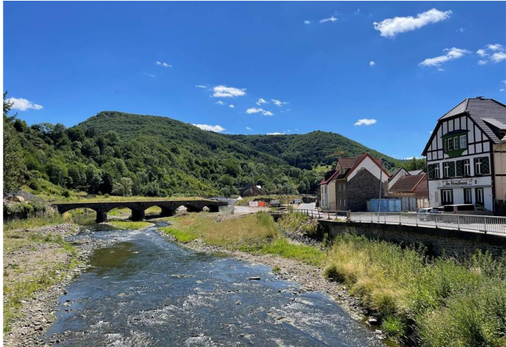
Condition before the flood disaster.
