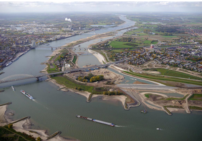
Condition after the measures.
