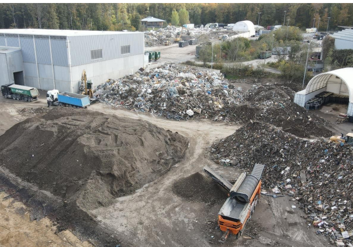
Construction waste phase.
