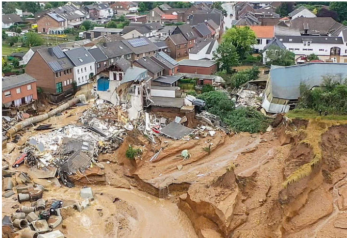
Condition after the flood disaster.
