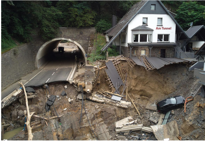
Condition after the flood disaster.
