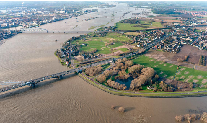
Condition before the measures.
